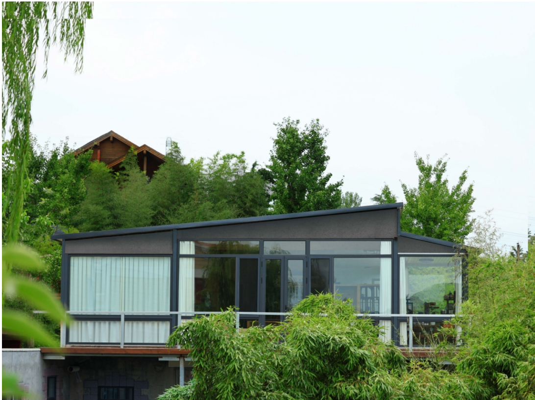
Figure 7.1: On-site photograph of the extension
